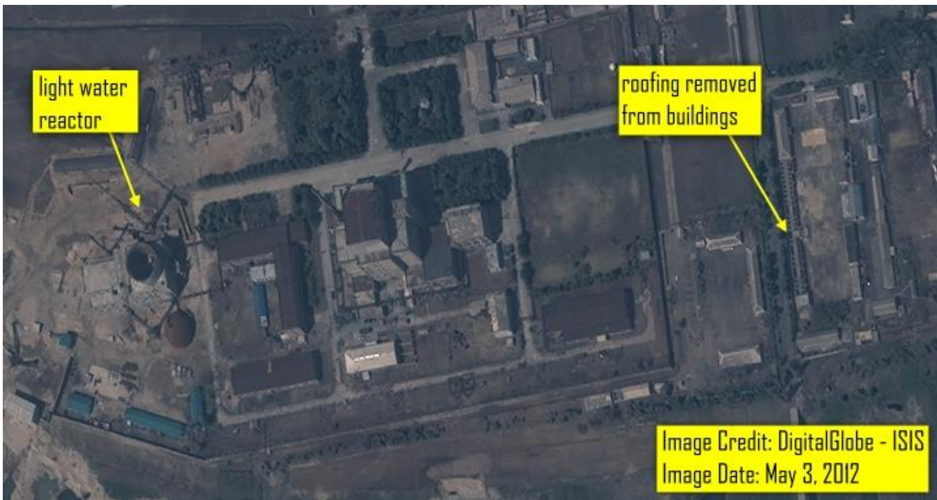
Figure 4. A wide area view of the Yongbyon LWR complex showing ongoing construction work on two buildings north of the reactor building.
