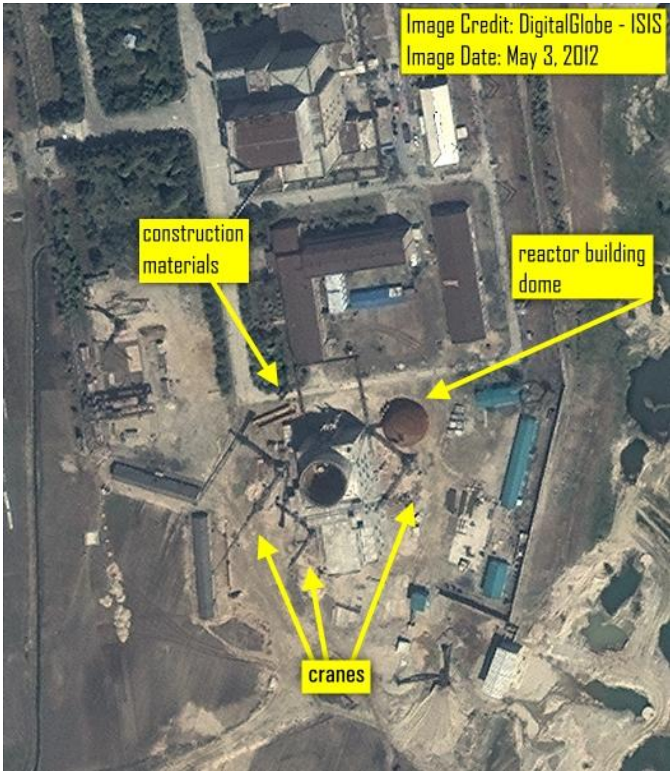
Figure 1. Satellite imagery from May 3, 2012 showing construction materials and support equipment waiting to be placed on the reactor building.
