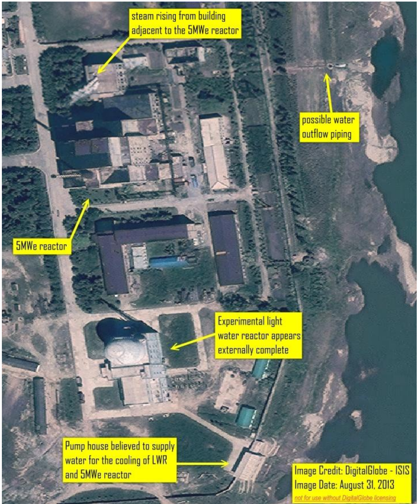
Figure 1. DigitalGlobe imagery showing the venting of steam from a building adjacent to the 5MWe reactor indicating that the reactor might have restarted operation.
