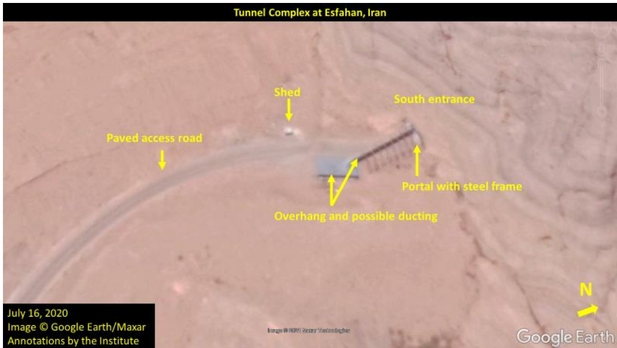
Figure 7. The South entrance tunnel as of July 2020.
