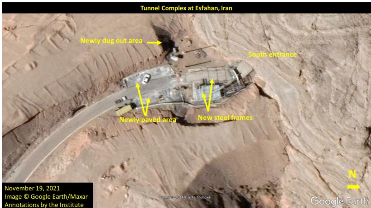
Figure 8. The South entrance in November 2021 after a year of construction activity.
