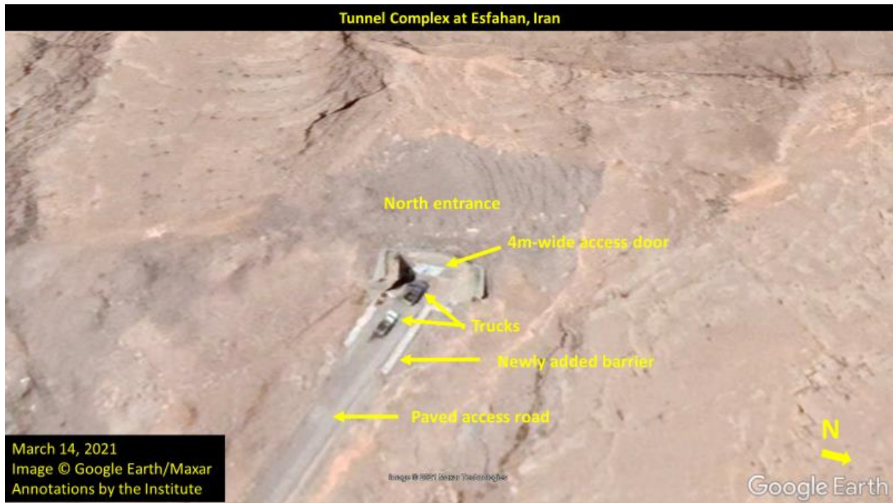
Figure 3. The North entrance tunnel in March 2021, shortly after construction activity began at this tunnel entrance, which has remained unchanged for many years.
