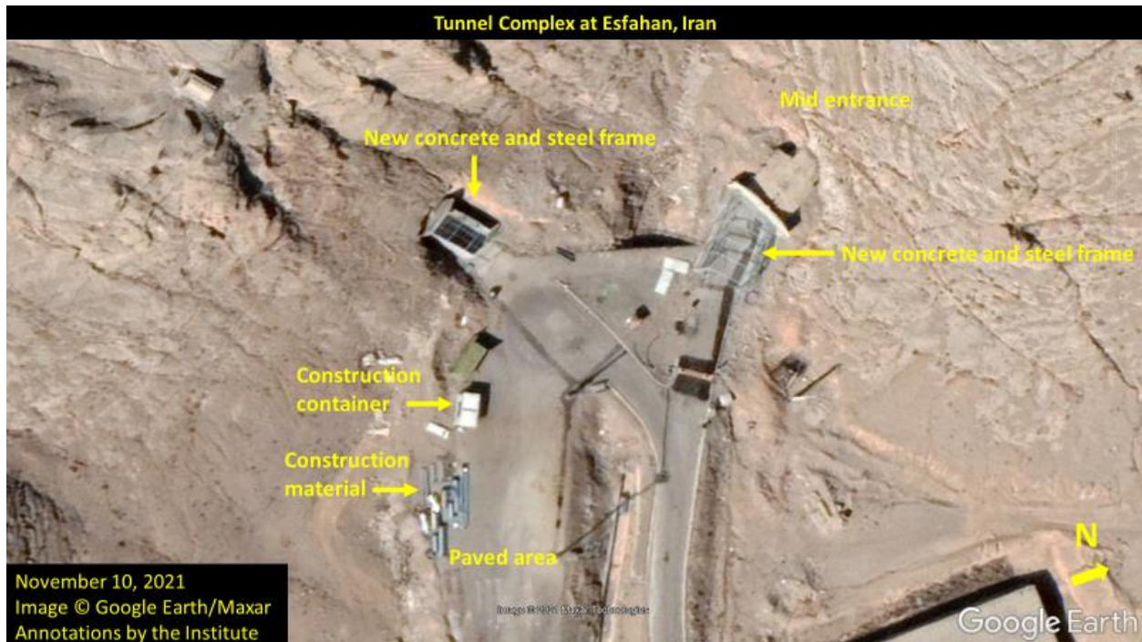
Figure 6. The two underground portals in the mid-entrance area in November 2021 after construction activity.
