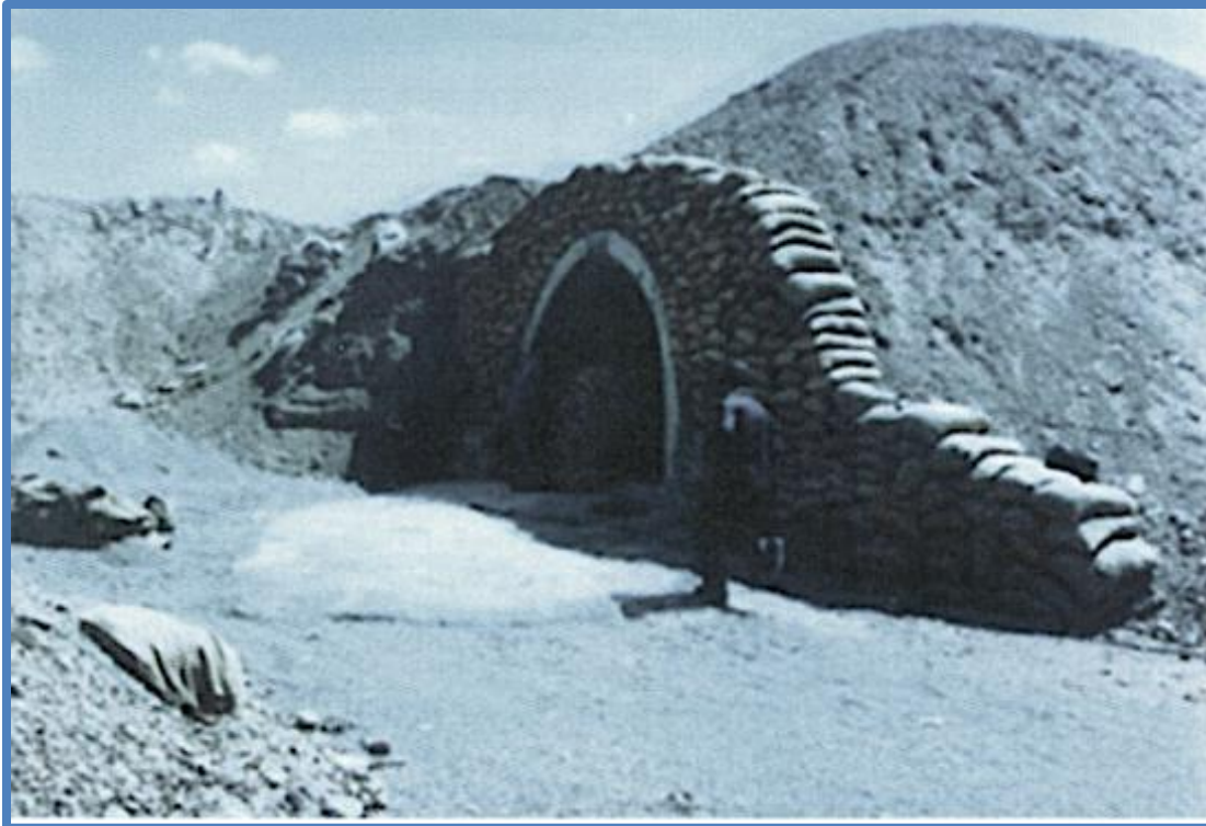
Figure 3. A ground photo from the Nuclear Archive shows the entrance area of the main bunker.
