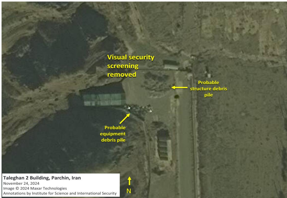
Figure 7. Later in November, the demolished building remains covered, but the visual security screening is removed.
