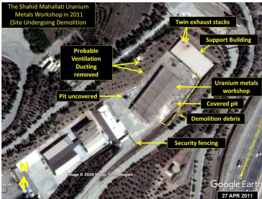
Figure 16. Extensive removal and demolition work is visible in an April 27, 2011 Google Earth image.
