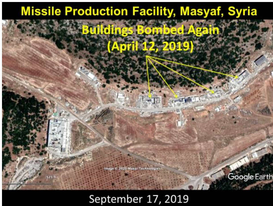
Figure 5. Several of the buildings were bombed again in April 2019. The damage can still be seen in this September 2019 image.
