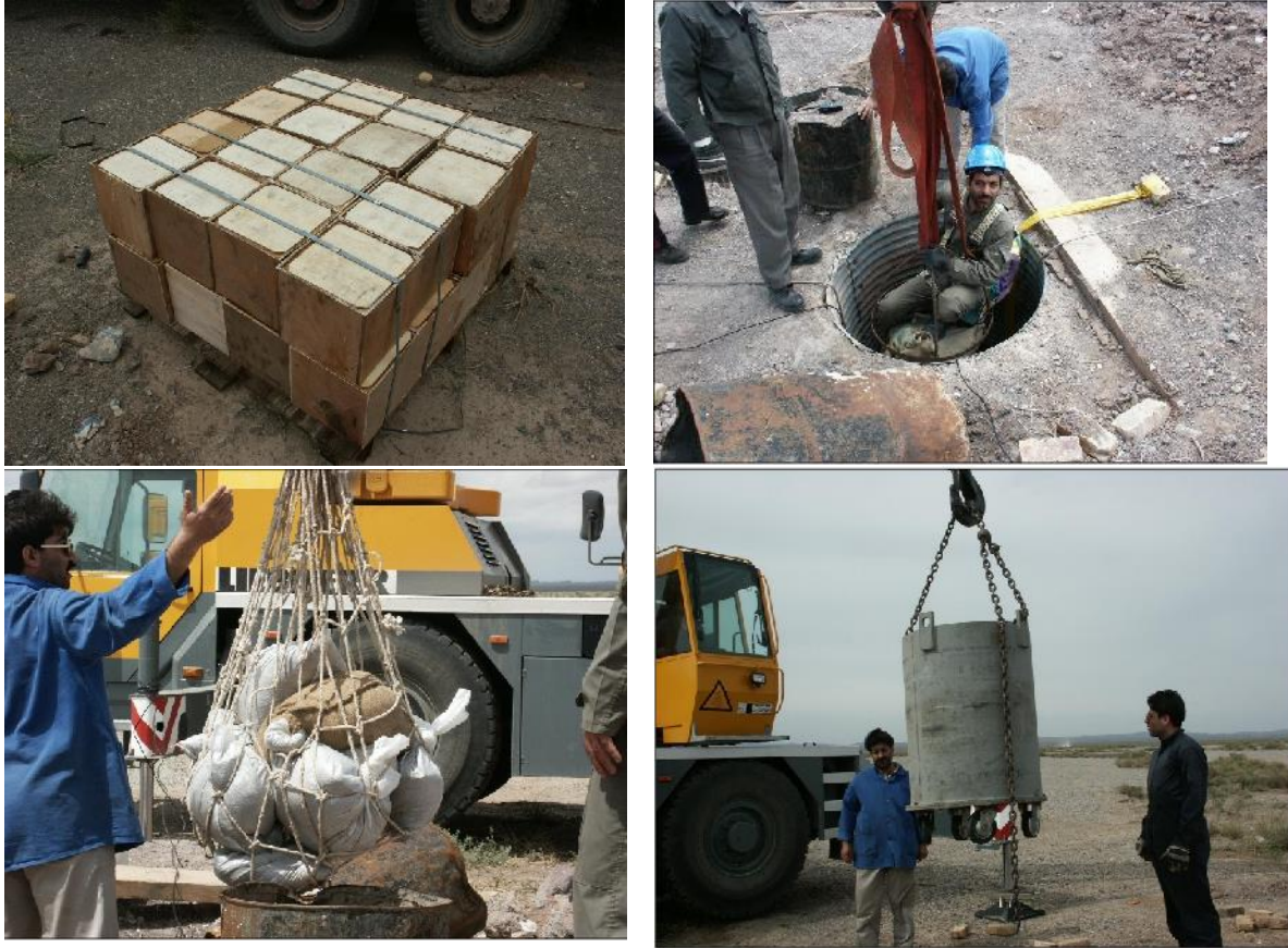
Figure 22. Archive images of high explosive tests. High explosives in upper left image. High explosive shaft (upper right). Possibly fill material for the shaft (bottom left) and capping it with a concrete plug, prior to detonation (bottom right).
