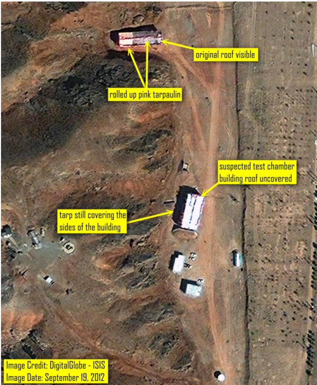
Figure 1: September 19, 2012 imagery showing the pink tarpaulins that previously covered the buildings being rolled back. There are no signs of construction of the terrace/wall or of the dirt piles that appear in later imagery.
