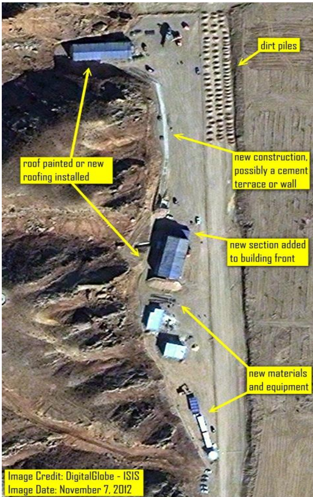
Figure 2: The latest image from DigitalGlobe clearly showing the new blue roofing of the two major buildings, new equipment and materials and the rows of earth piles. Numerous cars present at the site suggest a considerable level of activity at the site.
