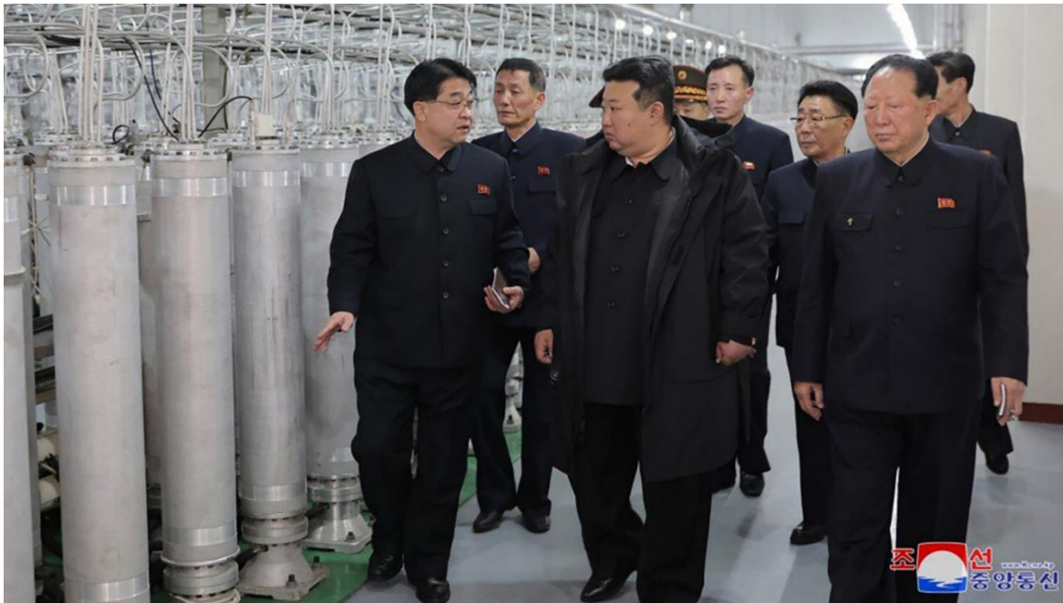
Figure 22. Two views of a long cascade hall in a low-roofed building, likely the Yongbyon Enrichment Plant Annex built in about 2022. The silver cabinets have wires running from them. Wire conduits are visible with wires running to individual centrifuge motors. Electro-pneumatic valves are visible on the dump line. Also visible are pressure gauges and vibration detectors. In addition, on the upper image the feed and product pipe can be seen exiting the cascade and returning to a central station. The feed point(s) cannot be identified. The pressure gauges in the images, which are on the top caps, look more cylindrical and could be pressure transducers.
