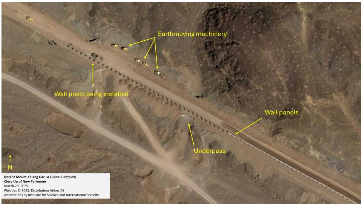
Figure 5. A close up of wall panelling underway.
