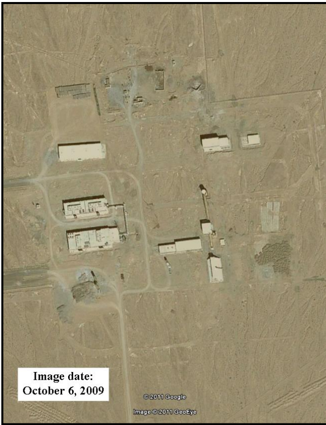
Figure 5. Ardakan yellowcake production facility under construction in this October 6, 2009 satellite image.
