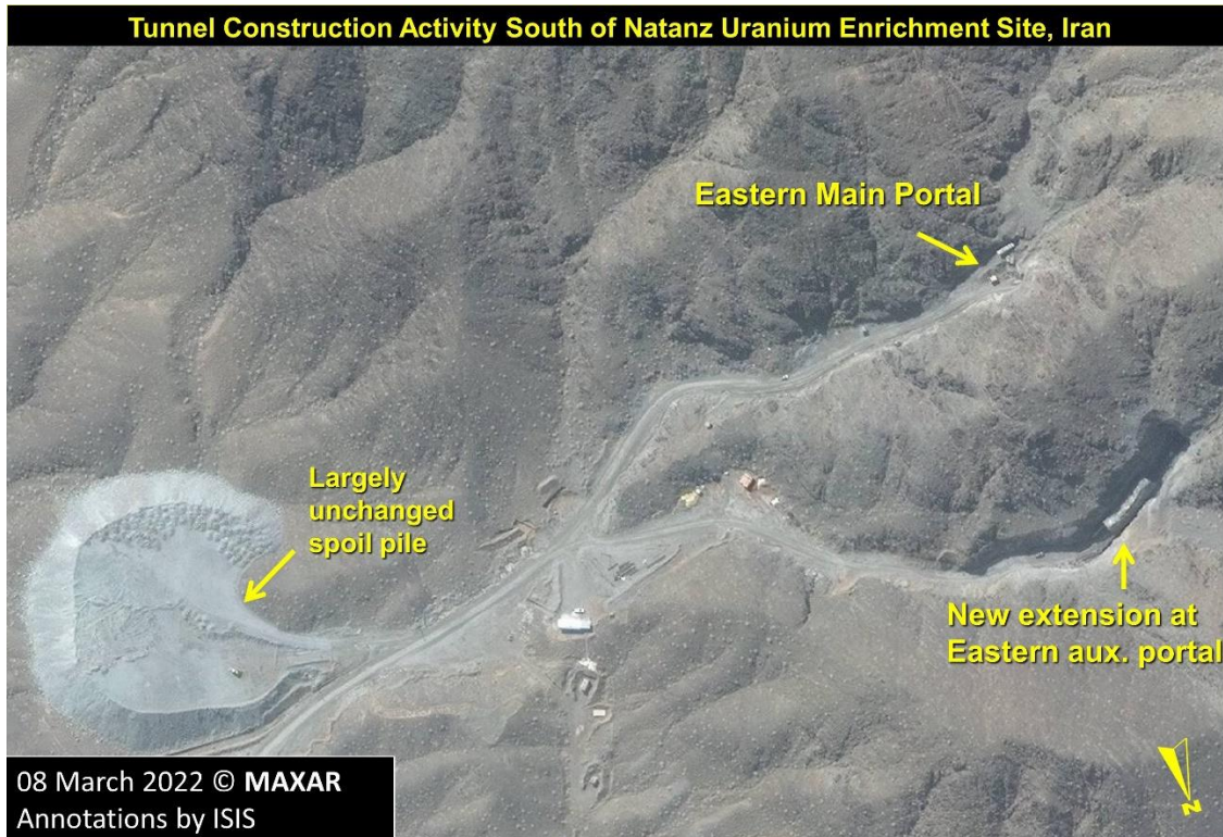
Figure 2. One of the two eastern tunnel portals shows a likely permanent tunnel entrance extension, adding further protection to the entrance.
