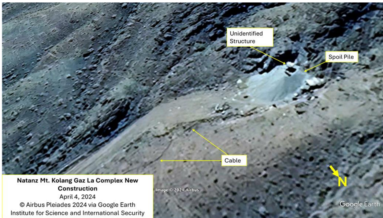
Figure 3. The construction site for a probable ventilation shaft on April 4, 2024.
