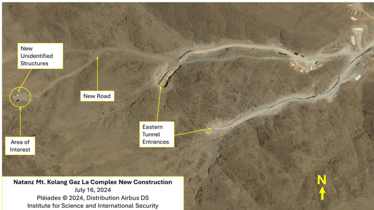
Figure 5. The construction in the latest imagery available on July 16, 2024, compared to the location of the two Eastern Tunnel Entrances.
