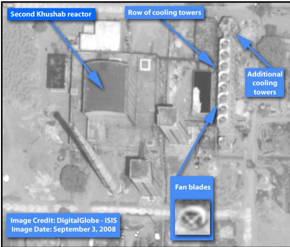
Figure 4. Close-up view of row of cooling towers with construction of additional cooling towers. The fan blades of the mechanical draft cooling towers can be seen.
