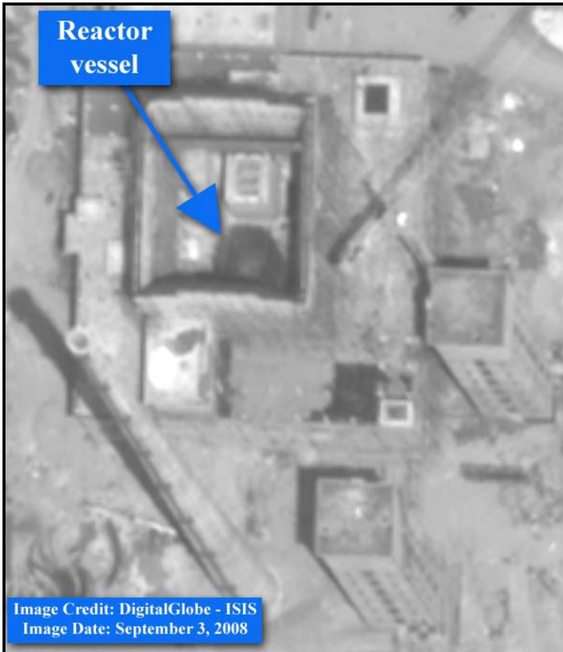
Figure 2. Third plutonium production reactor at Khushab.
