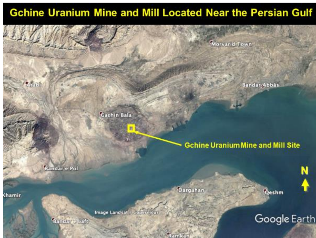
Figure 1. Gchine uranium mine and yellowcake production plant, or mill, in southern Iran.
