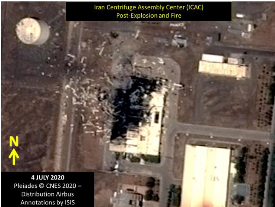
Figure 2. The ICAC Building as it appeared in this July 4, 2020 CNES/Airbus satellite image acquired the day after the explosion and fire.
