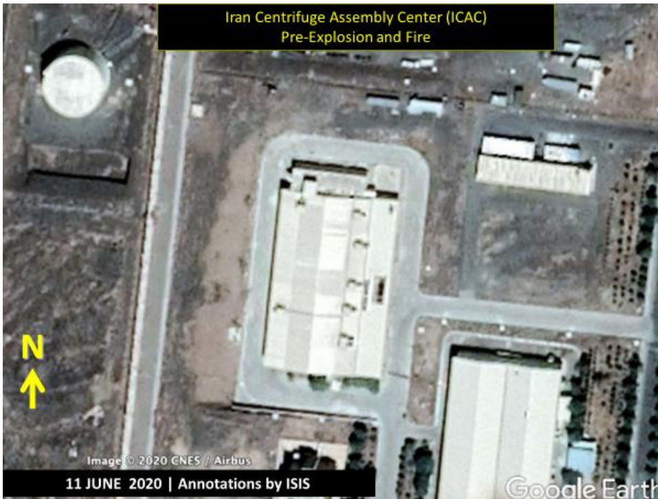
Figure 1. The ICAC Building as it appeared in this June 11, 2020 CNES/Airbus satellite image as found on Google Earth.
