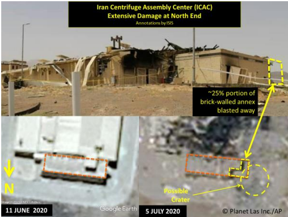
Figure 7. The top ground image is of the north end of the ICAC Building as published by the Atomic Energy Organization of Iran as it appeared following the explosion and fire showing where a section of the annex was blasted away. The lower left image is from Google Earth and shows the appearance of the 30 meter long annex pre-incident, while the lower right image of the annex from July 5, 2020 (as published by CNN) shows by comparison that approximately 25 percent of the annex was blasted away, as well as its proximity to the possible crater.
