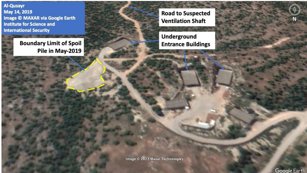
Figure 2. This shows the size of the spoil pile that is near the upper tunnel entrance building in May 2019.
