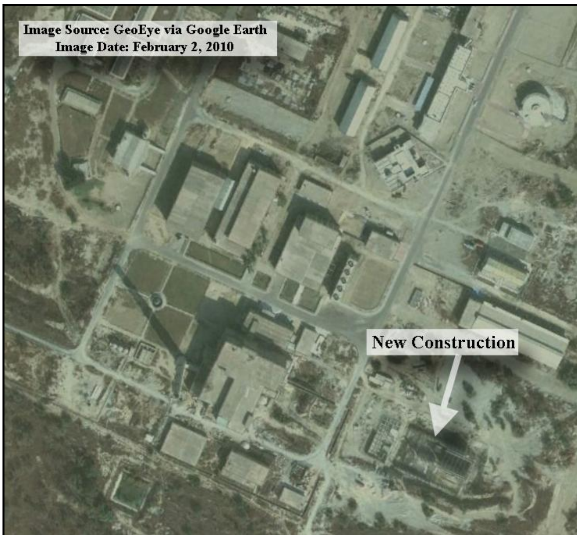
Figure 4. February 2, 2010 image showing continuing construction activity at a compound in the southwest corner of the Chashma site. ISIS speculated in a 2007 report that this was the site of the previously abandoned Chashma reprocessing plant. This compound appeared overgrown and unused in satellite imagery from 2000, but a resurgence of construction activity can be seen in the years that followed. For more on this compound, see the 2007 ISIS Report, " Chashma Nuclear Site in Pakistan with Possible Reprocessing Plant. "
