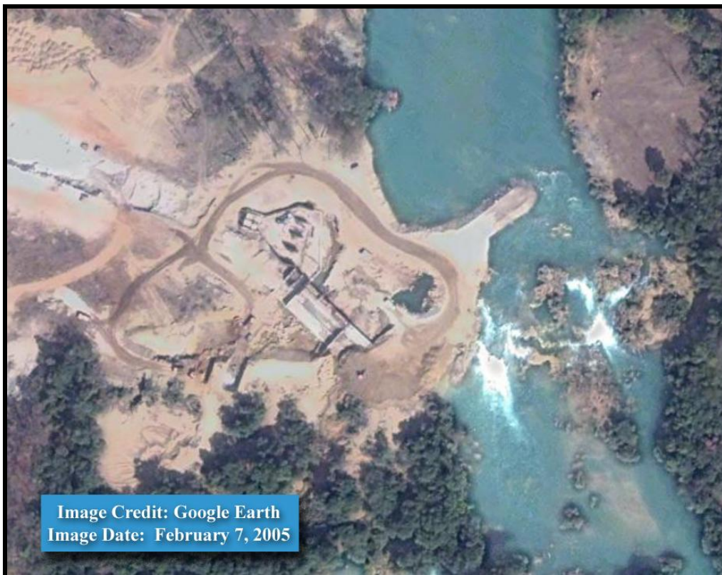
Figure 2. Example of dam construction located in Burma at 20.598385, 98.292722.
