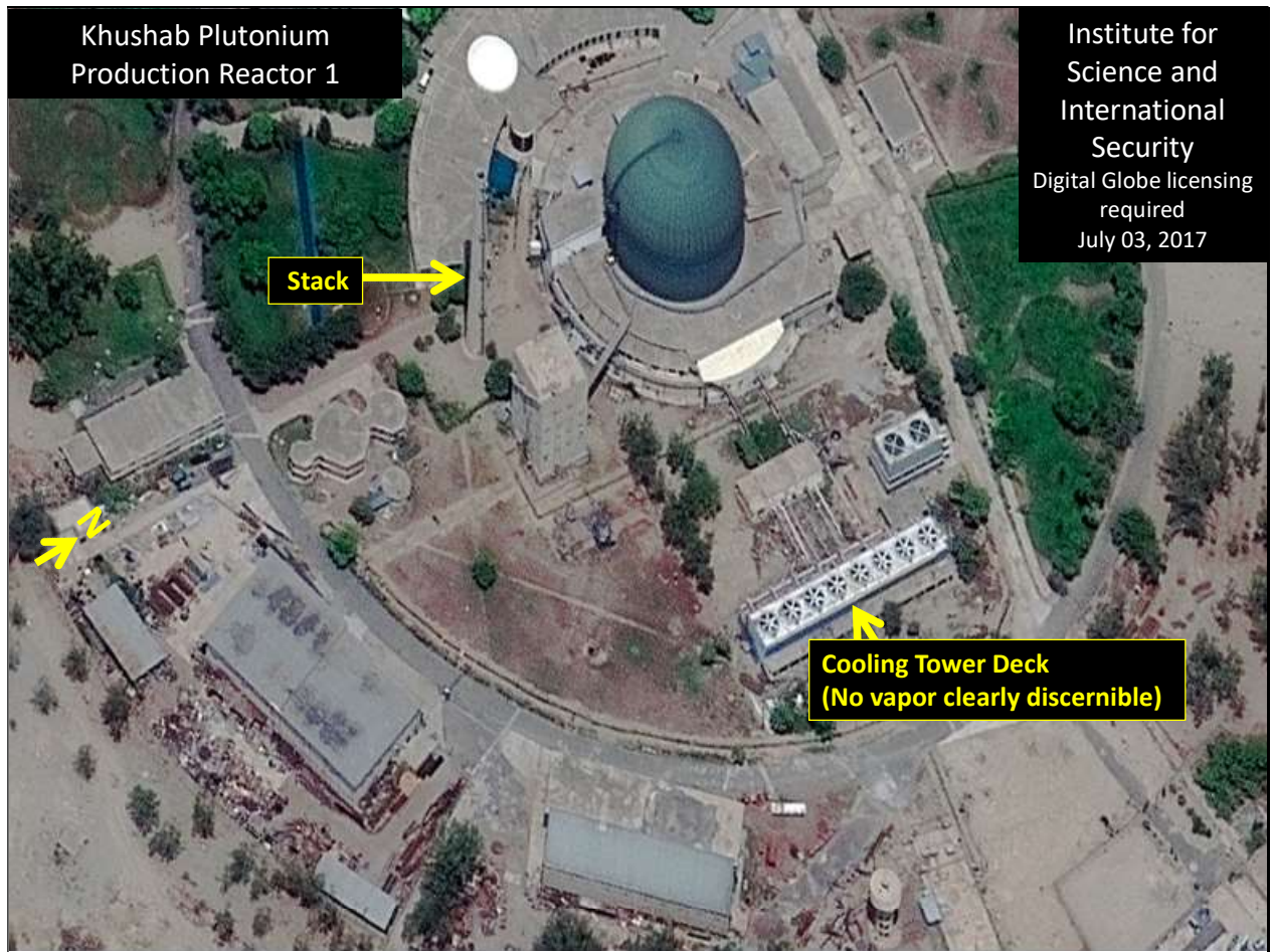
Figure 7. No vapor is visible coming from the cooling towers of Khushab 1.
