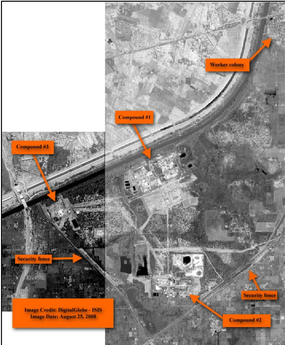
Figure 1. An overview of the Dera Ghazi Khan nuclear site in Pakistan. The site is made up of three main compounds, and the entire facility is surrounded by security fencing with intermediate guard stations. The worker colony is adjacent to the north-east section of the nuclear facility.
