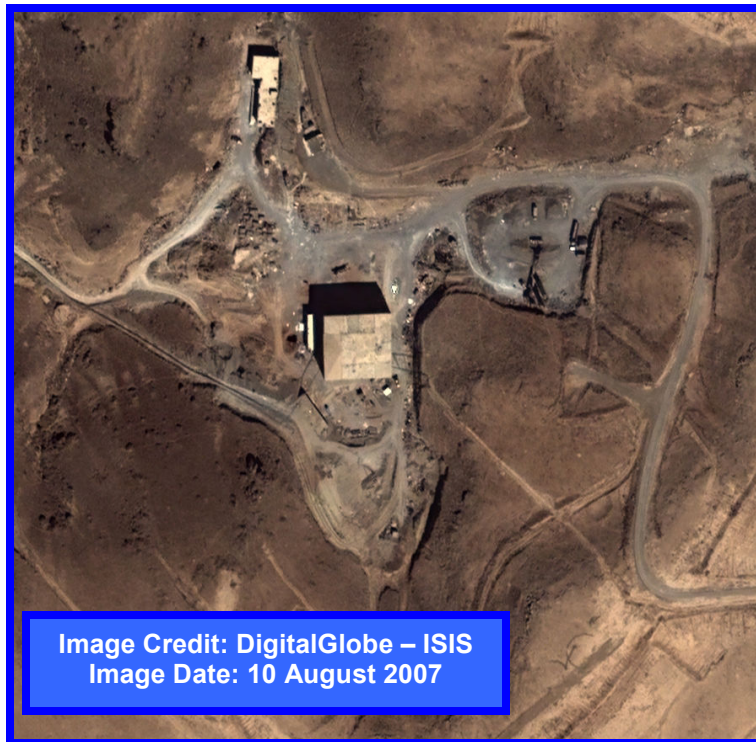
Figure 1. Overview of suspected reactor site before September 6, 2007
