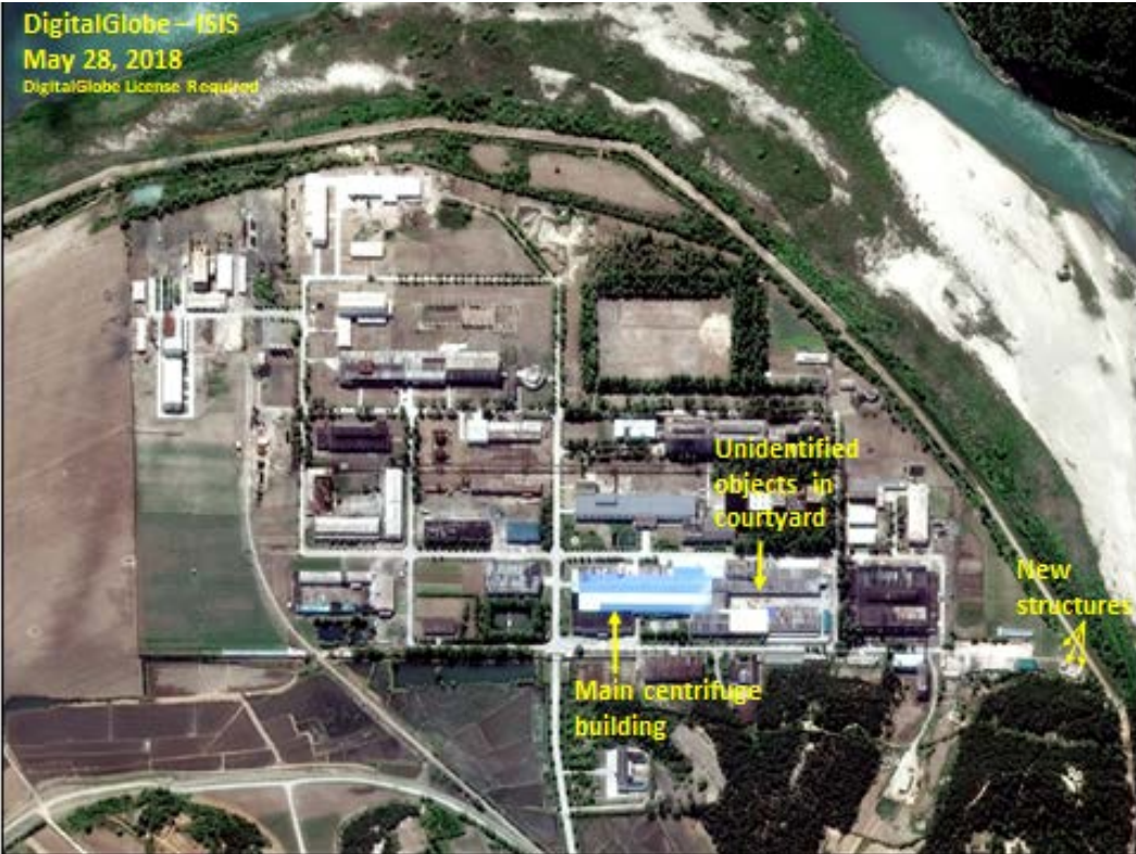
Figure 7. The fuel fabrication facility hosts the main centrifuge building.
