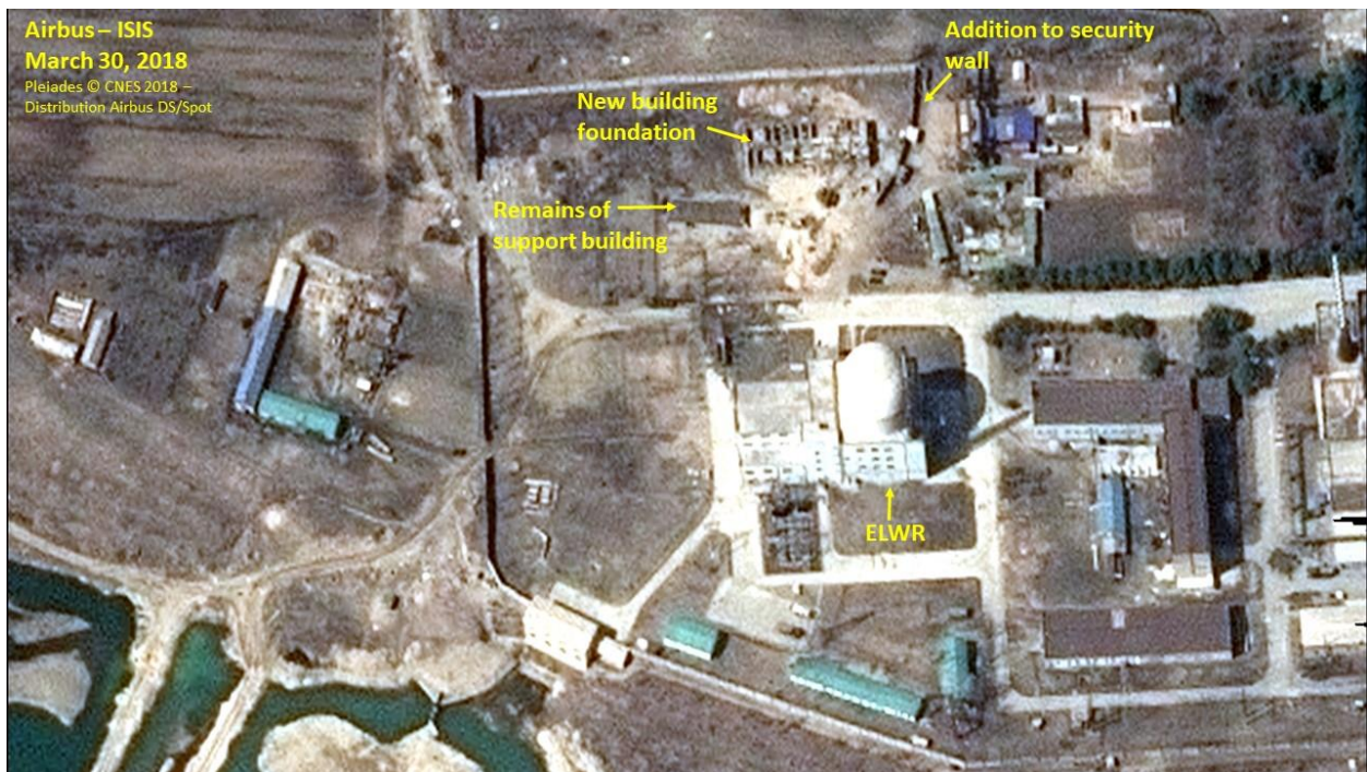
Figure 7. Construction of a new building is taking place near the ELWR. However, it is unlikely that the building is critical for reactor operation or an indication of when the reactor may commence operation.
