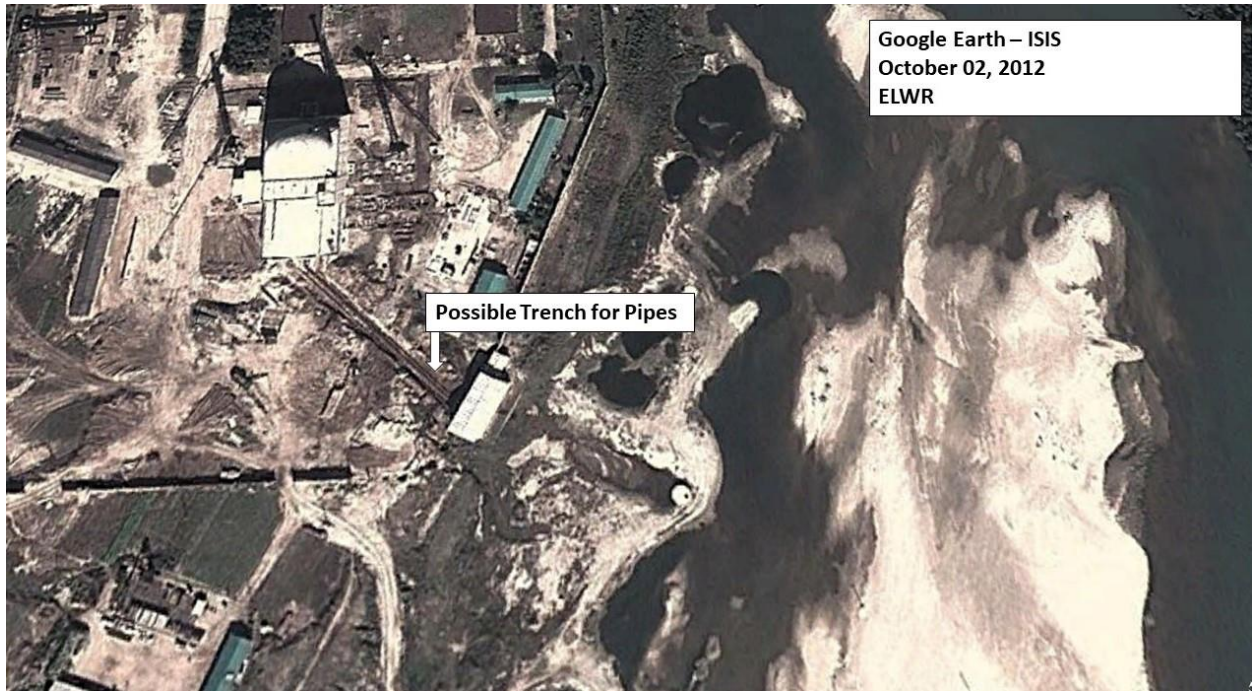
Figure 6. Possible pipe work in 2012 is one of the main indicators that the building by the river is a pump house or otherwise part of the ELWR's secondary cooling system.
