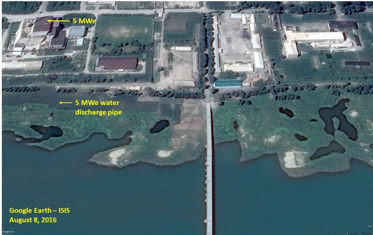
Figure 2. The riverbank and the water discharge pipe in 2016.
