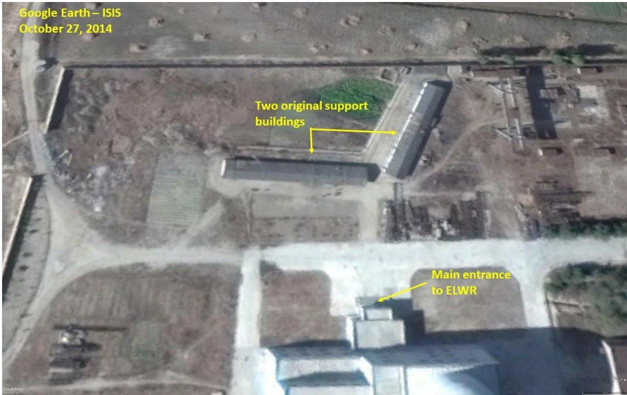
Figure 8. Two support buildings used to be located where construction of a new building is currently taking place.
