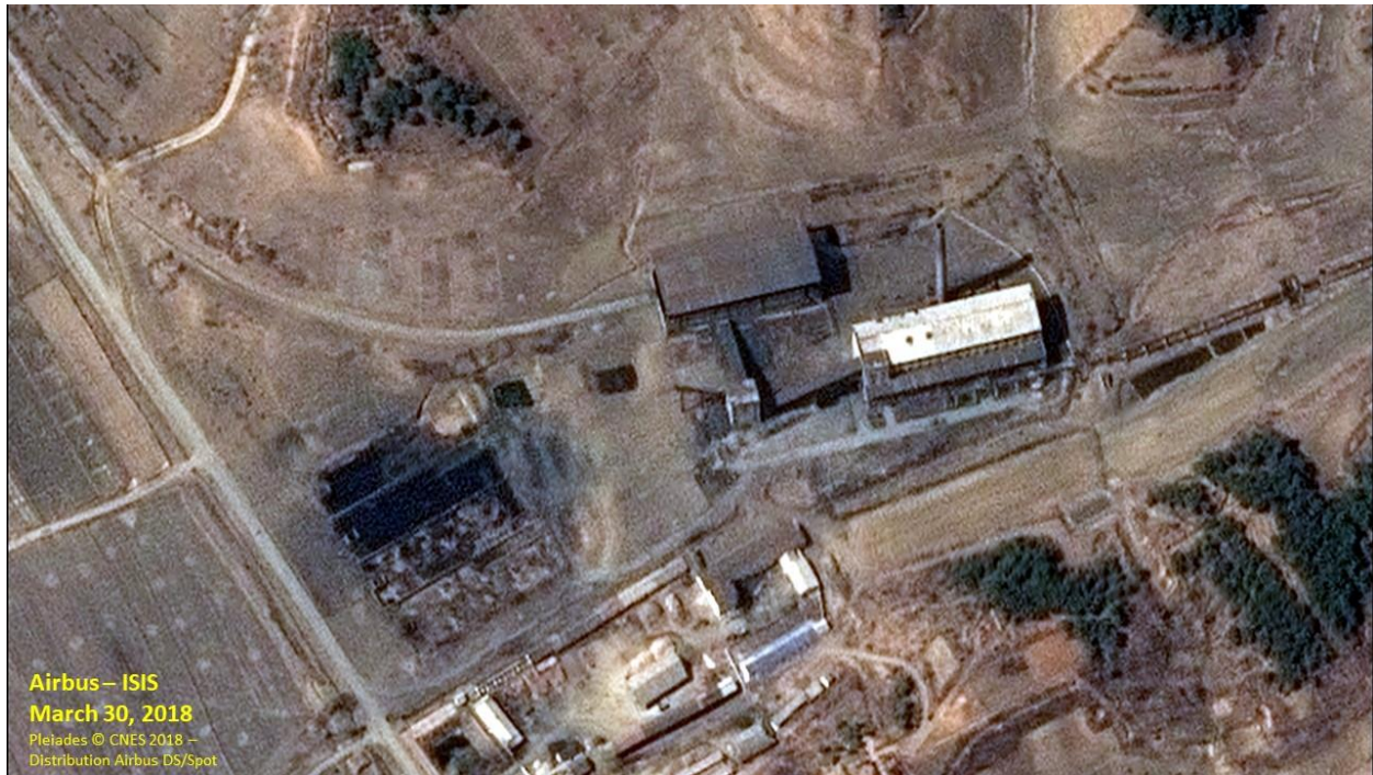
Figure 4. The coal-fired steam generation plant shows no visible signs of activity.
