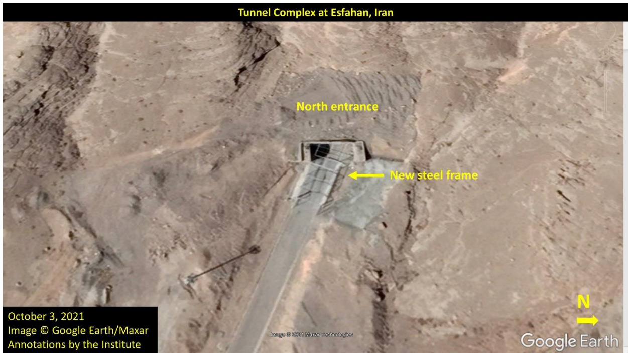
Figure 4. The North entrance tunnel in October 2021, after a steel frame was added to the entrance area.
