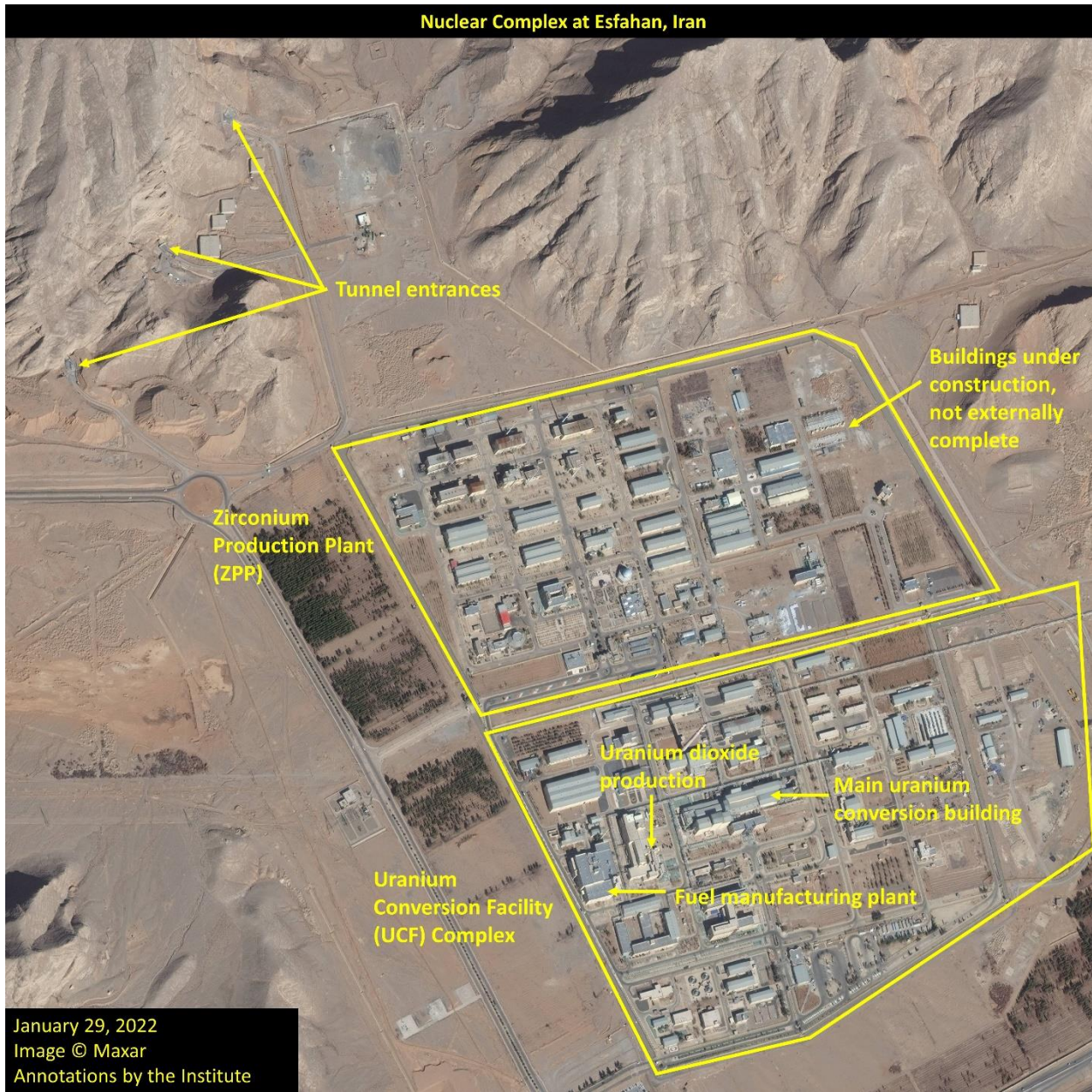
Figure 1. Overview of the Esfahan nuclear site in Iran, which includes the Uranium Conversion Facility (UCF) complex, Zirconium Production Plant (ZPP), and a tunnel complex. (In the Zirconium Production Plant area, there is also a building which features the logo of a company associated with uranium metal production.)
