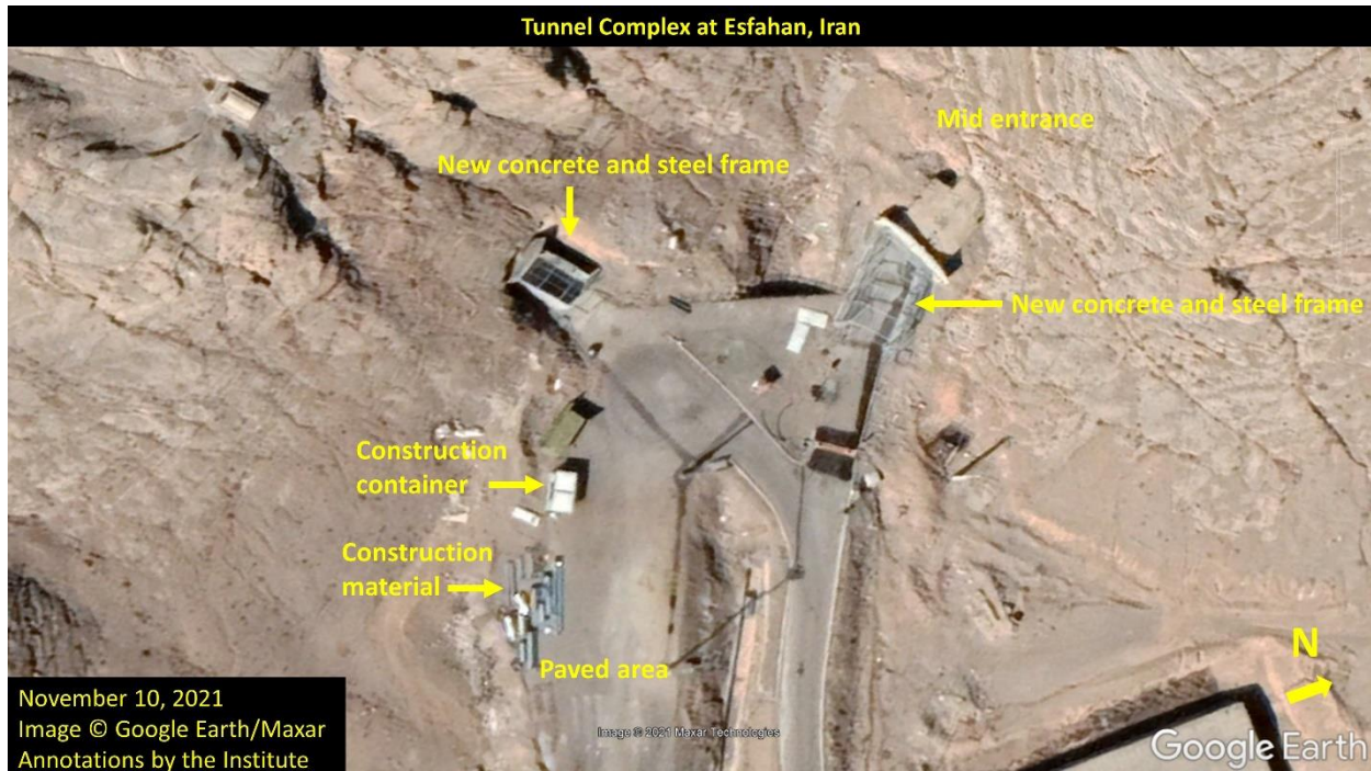
Figure 6. The two underground portals in the mid-entrance area in November 2021 after construction activity.
