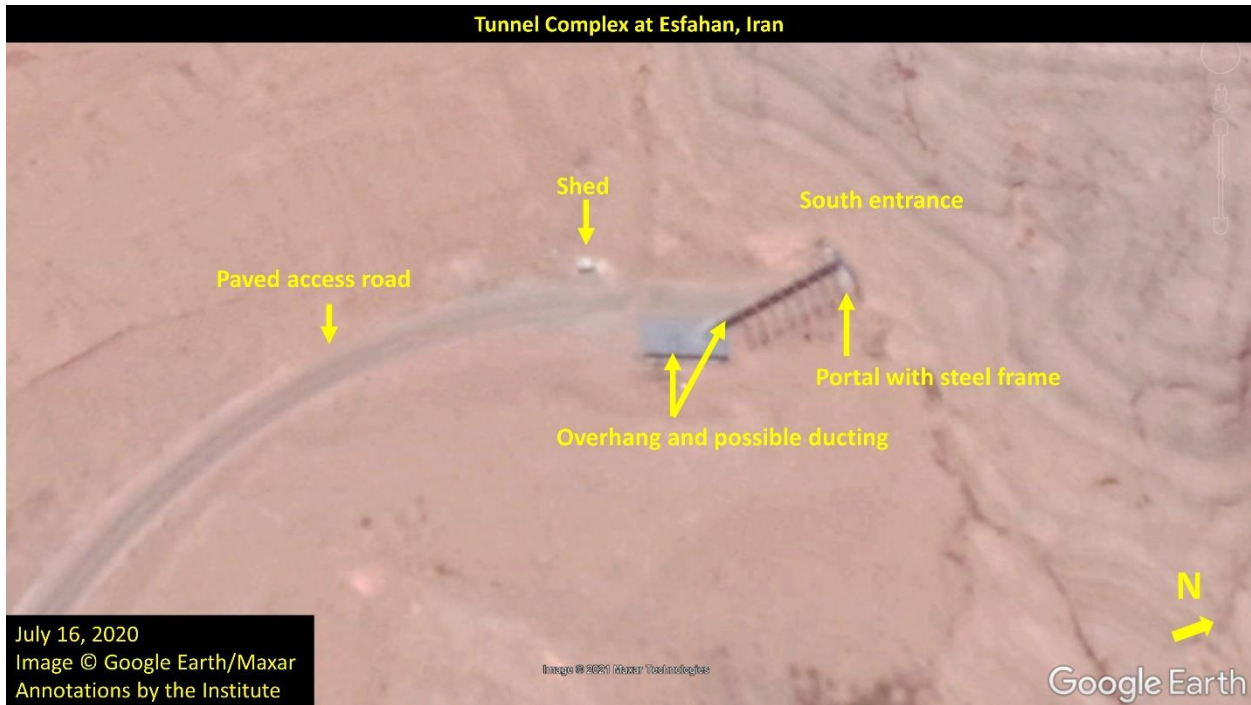
Figure 7. The South entrance tunnel as of July 2020.
