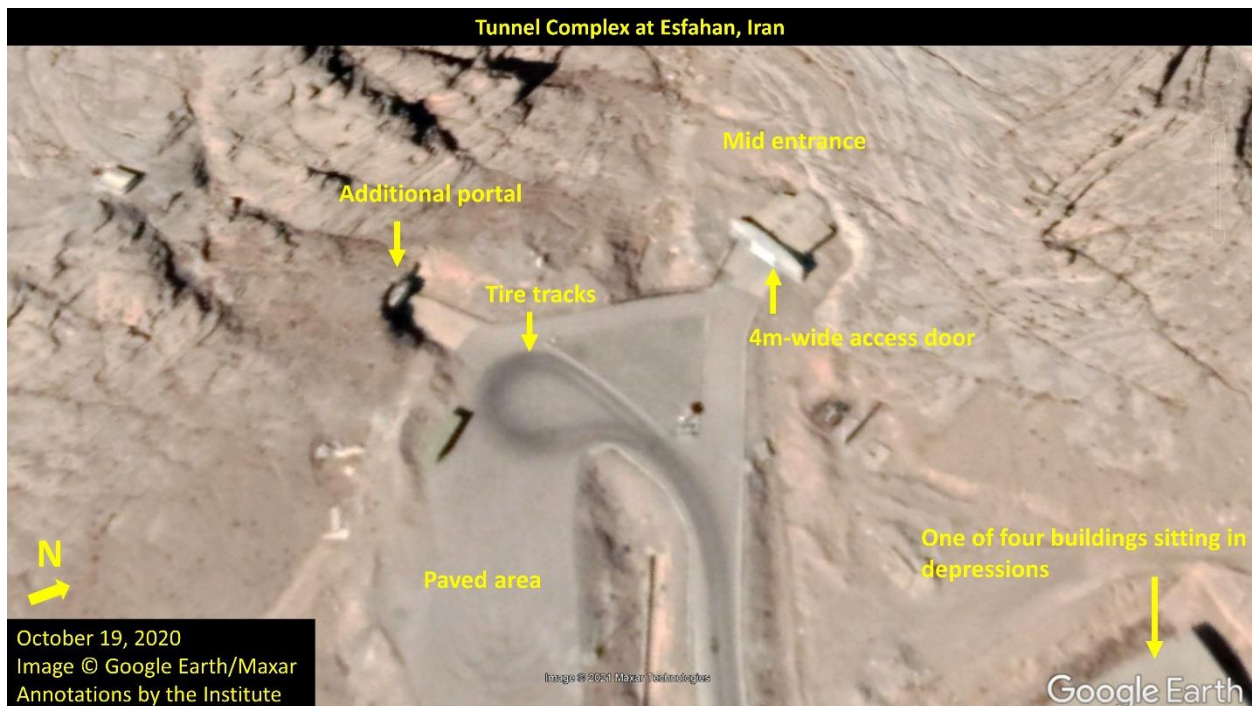
Figure 5. The two underground portals in the mid-entrance area in October 2020.
