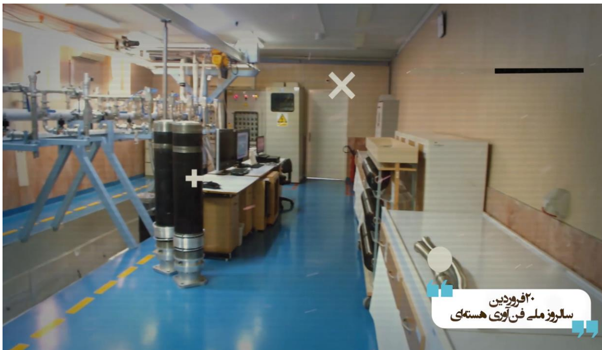
Figure 15. The video shows preparation for the installation of the centrifuge test stands in a testing pit. In the top photo, visible is the base flange of the centrifuge which will be bolted to the floor. The two IR-6 centrifuges in the bottom photo are awaiting lowering into the test pit, located to the left. Three rotor assemblies are visible along the right wall. The outer casings appear to be made of carbon steel rather than aluminum. Carbon steel casings have the advantage of being less expensive than aluminum ones, leading to frequent use in centrifuge programs, but carbon steel corrodes more easily, making aluminum preferable in Iranian enrichment plants.
