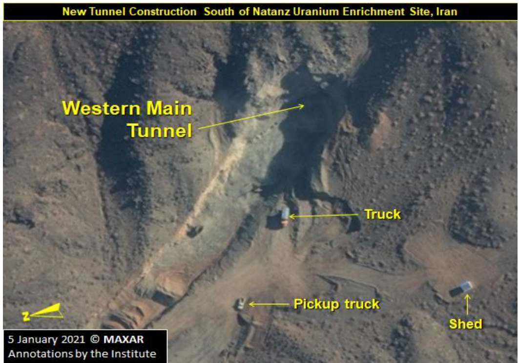
Figure 6. A close-up of the western main tunnel entrance.
