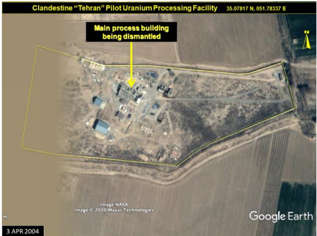
Figure 7. An image from April 2004 showing the dismantlement of the main building, consistent with IAEA reporting of building demolition having occurred in 2004.
