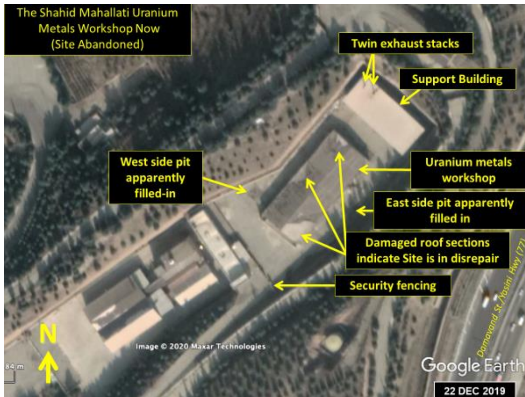
Figure 18. A recent Google Earth image showing apparently abandoned buildings
