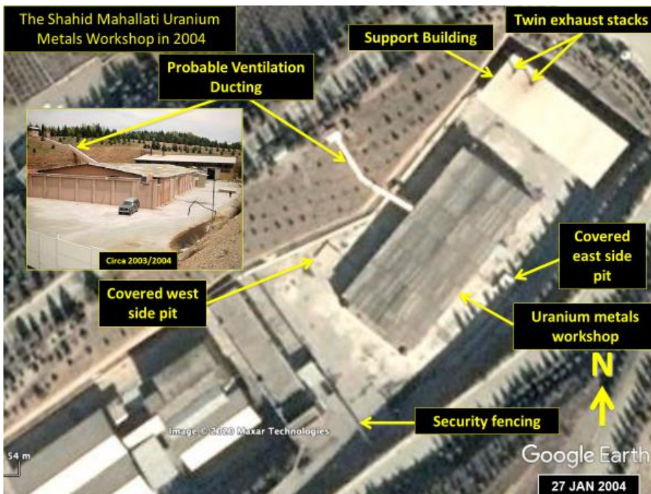
Figure 10. At top, a Maxar Technologies image from March 2003 (also shown in Figure 1). It shows the site mostly completed by this time, with the fence and ventilation duct in place, the pits covered, and only a few piles of rubble or equipment left outside. At bottom, a Google Earth image from January 27, 2004, of the uranium metals workshop, which correlates perfectly with the ground images from the Nuclear Archive as shown in the inset. The location of the fence opening matches the location of the gate visible in ground photos.
