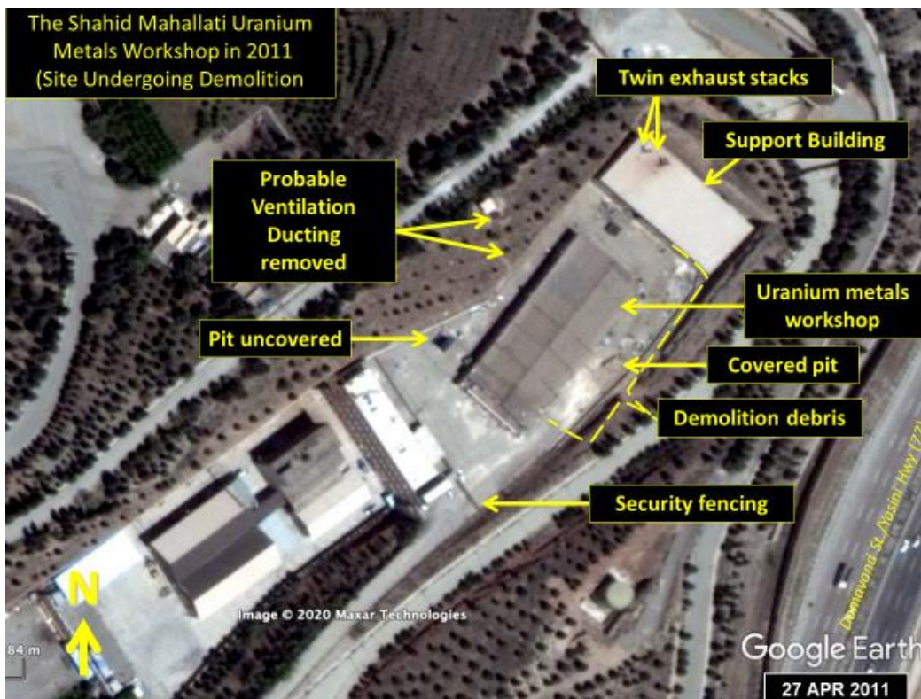
Figure 17. Extensive removal and demolition work is visible in an April 27, 2011 Google Earth image.
