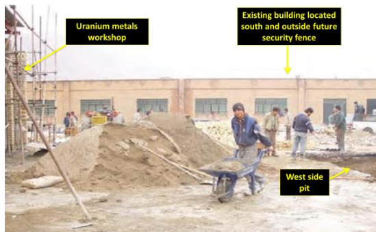
The Shahid Mahallati Uranium Metals Workshop Under Construction Circa 2002/2003
