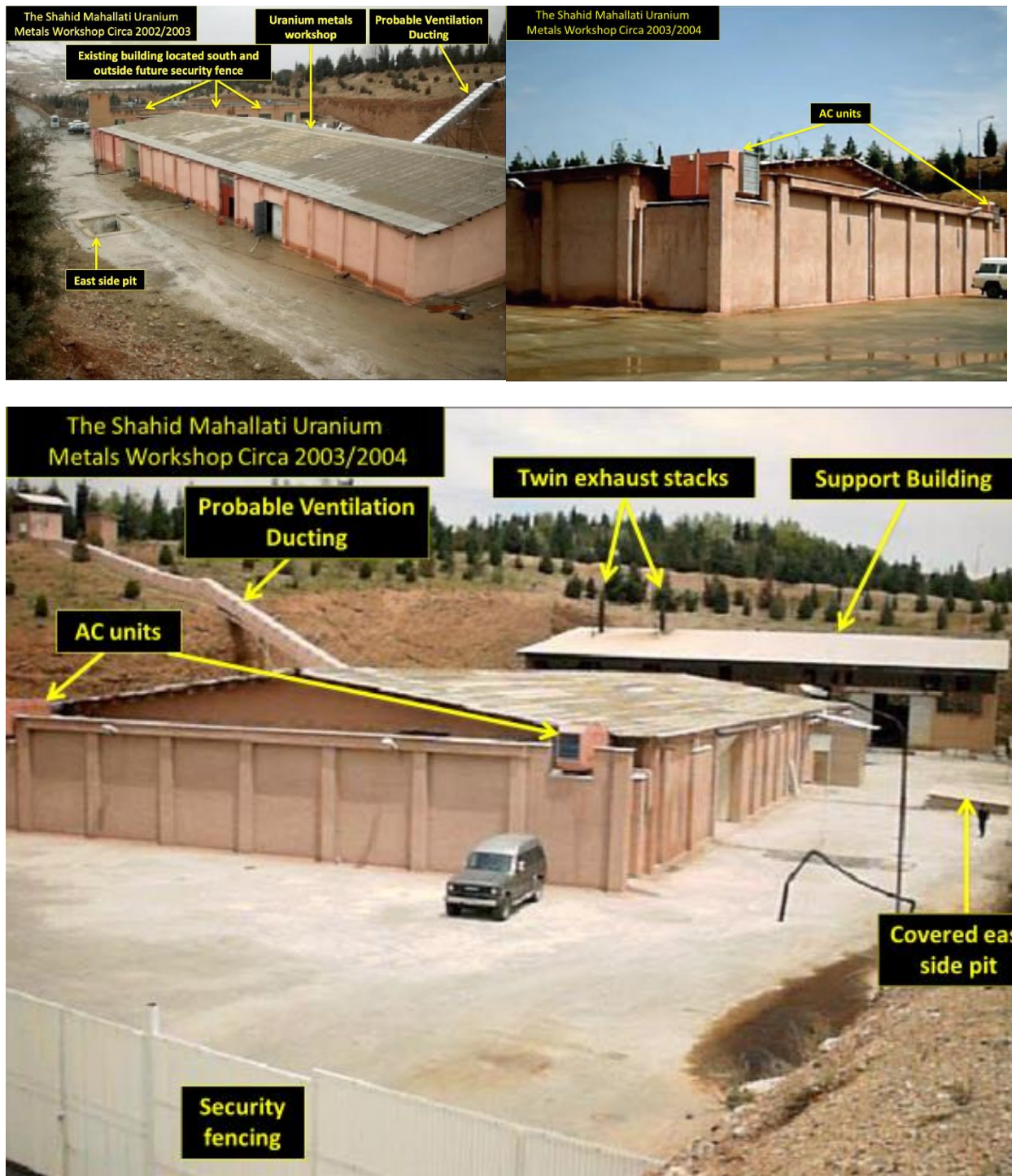
Figure 9. Nearly complete uranium workshop. Visible in upper images, metal ducting, two air conditioner (AC) units, and one of two pits without a cover; visible in lower image, a covered pit and a security fencing. All images from the Nuclear Archive, annotated by the Institute.
