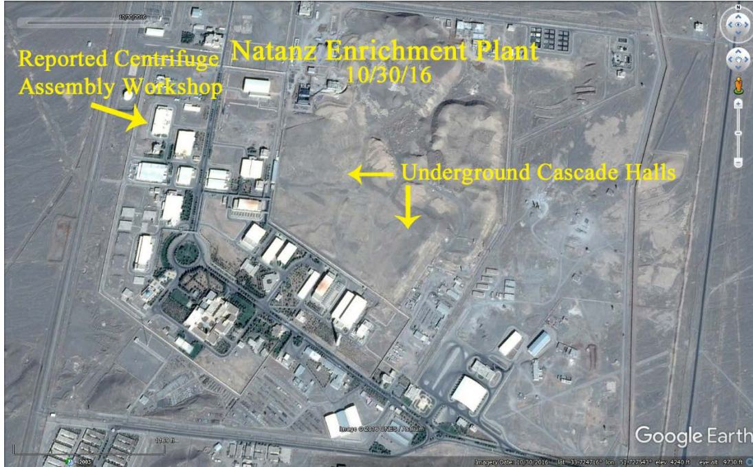
Figures 1-3: The Natanz enrichment site showing a reported new centrifuge rotor assembly workshop near the pilot enrichment plant. Early construction activities of this workshop can be seen in a 2012 image. The underground cascade halls of the Fuel Enrichment Plant are also nearby. Images courtesy Google Earth.
