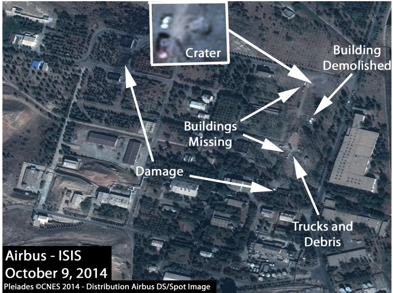
Figure 2. Airbus imagery dated October 9, 2014 showing the status of the site of the alleged explosion or fire at the Parchin military complex.
