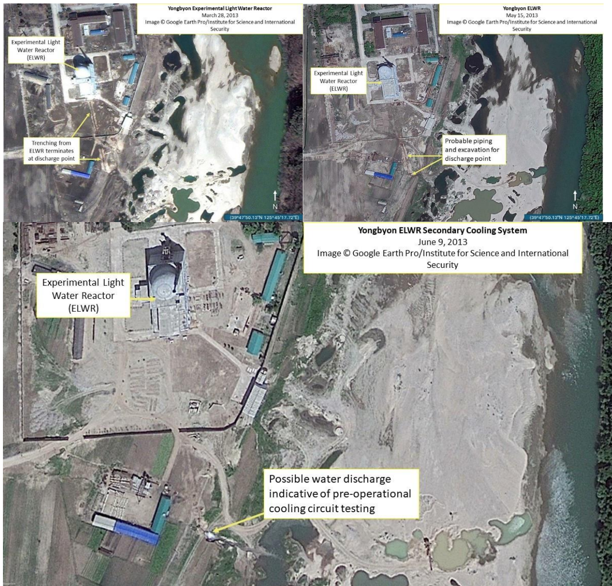
Figure 4. Trenching and excavation activities in 2013 show that the water discharge point is directly connected to the ELWR.
