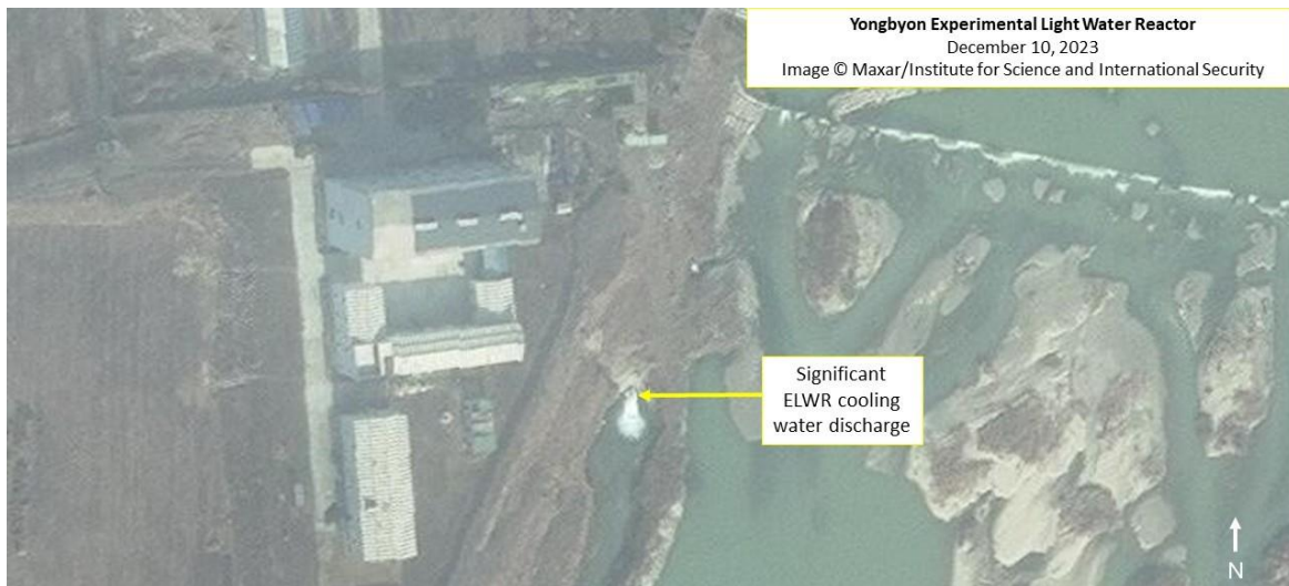
Figure 2. A December 10, 2023, image shows significant water outflow at the ELWR cooling water discharge point.
