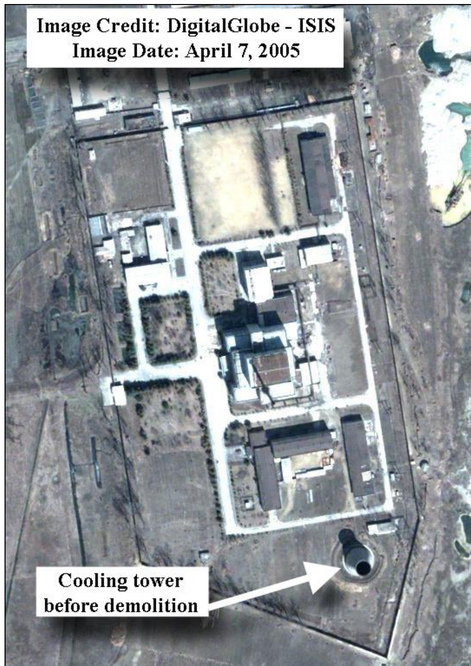
Figure 5. April 7, 2005 DigitalGlobe satellite image of the reactor site before the cooling tower was demolished
