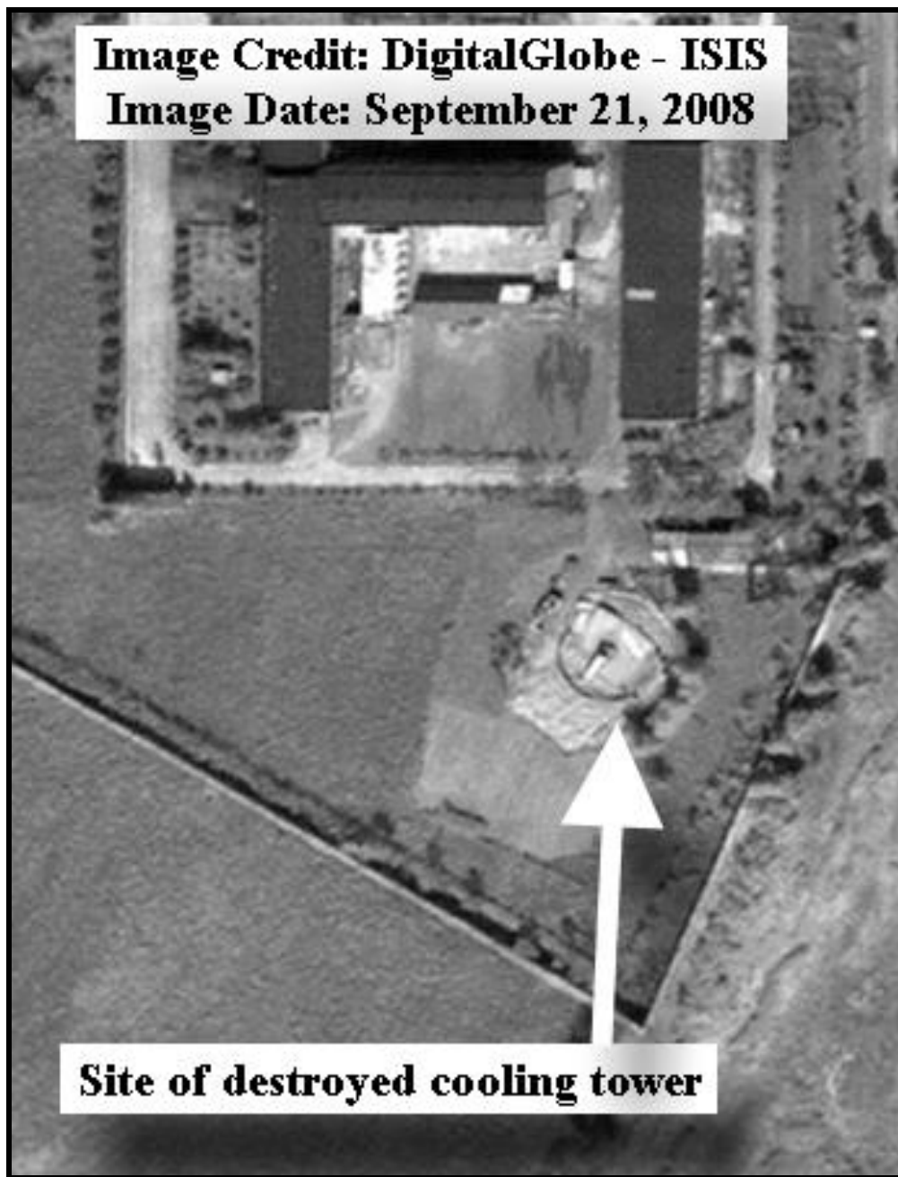
Figure 2. September 21, 2008 DigitalGlobe satellite image of the same site. Only the remaining foundation of the destroyed cooling tower can be seen.
