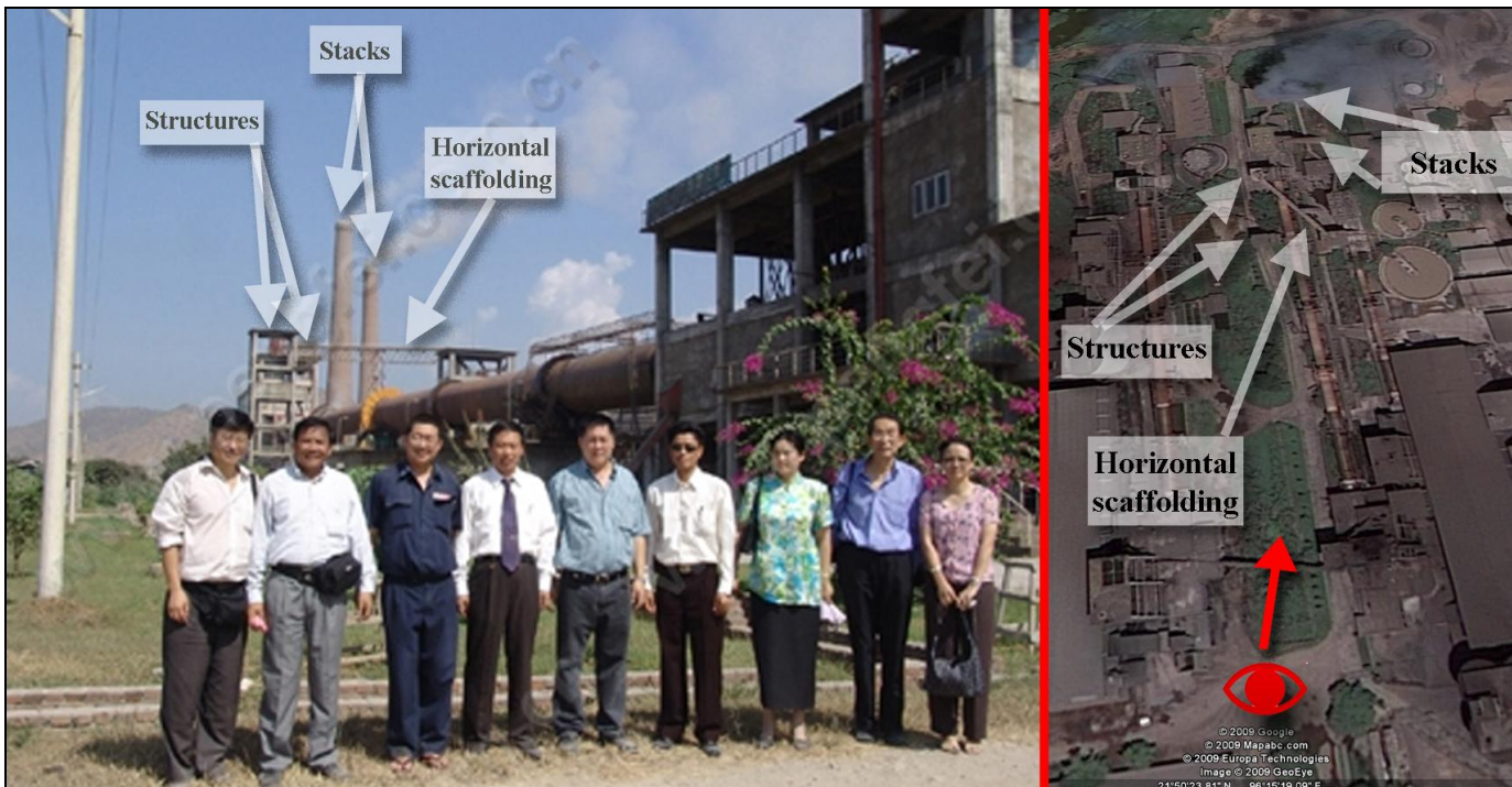
Figure 3. On the left, a ground photograph of the AAA Cement Plant in Myanmar 3 . On the right, a GoogleEarth satellite image of the Myit Nge Chaung site. The location of stacks, piping and structures appear to correspond between the two images.
