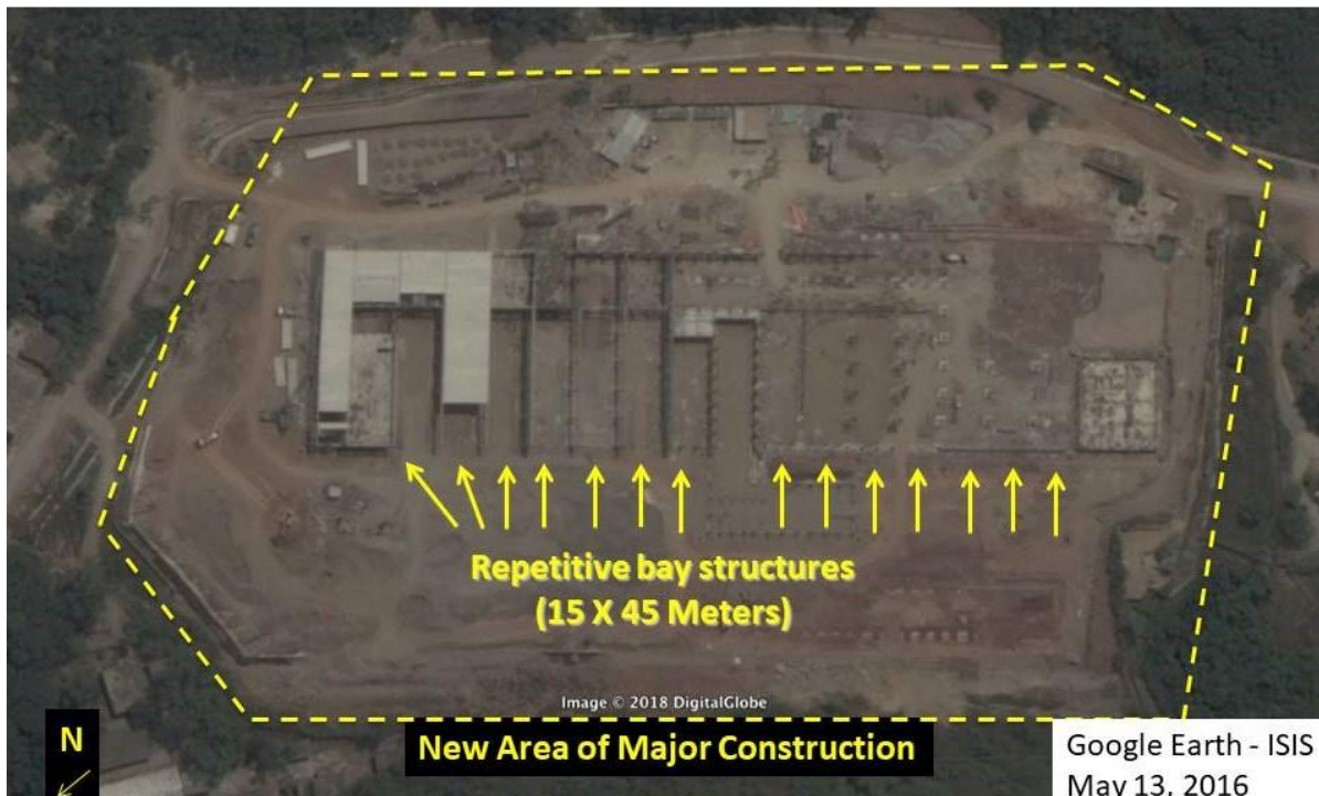
Figure 5. Construction showing the emerging bay structure.
