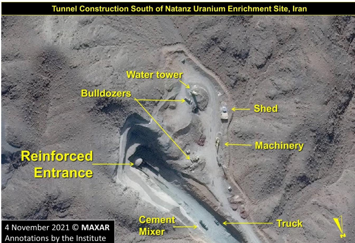
Figure 4. Close-up of the Western tunnel portal.
