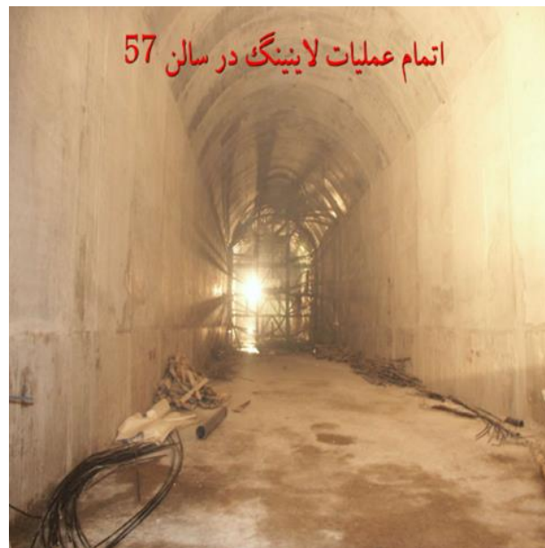
Figure 5. Iran Nuclear Archive tunnel schematic for Shahid Boroujerdi (rotated 90 degrees for easier viewing), along with archive images of the construction of the tunnels, showing lining of the tunnels.
