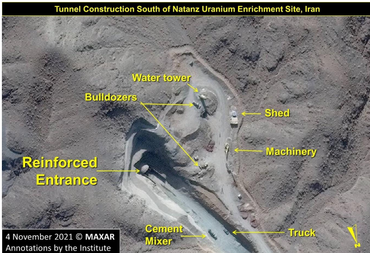
Figure 4. Close-up of the Western tunnel portal.
