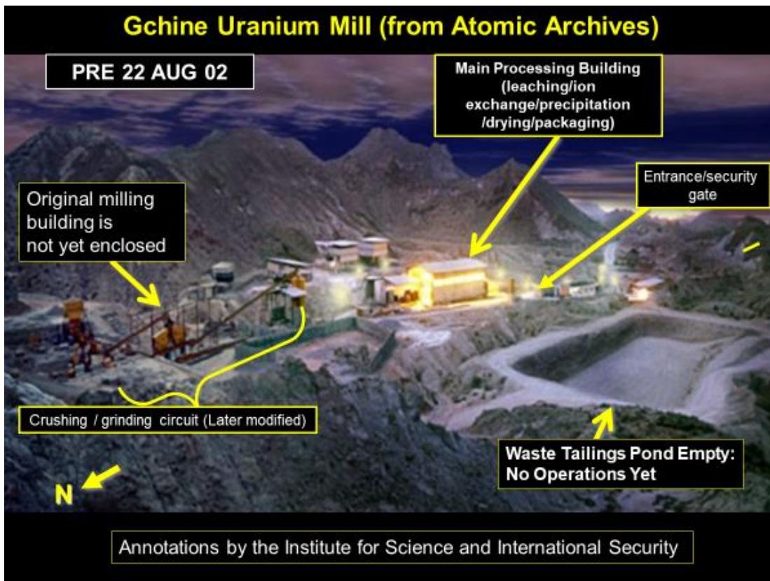
Figure 2. The Gchine yellowcake production plant, or mill, as seen in a photo discovered in the Iran Nuclear Archive (sometimes called the Atomic Archive.)
