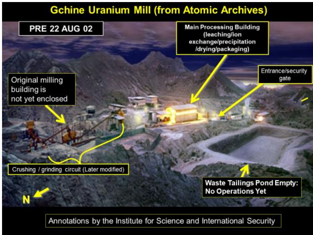
Figure 1. The Gchine yellowcake production plant, or mill, as seen in a photo discovered in the Iran Atomic or Nuclear Archive.
