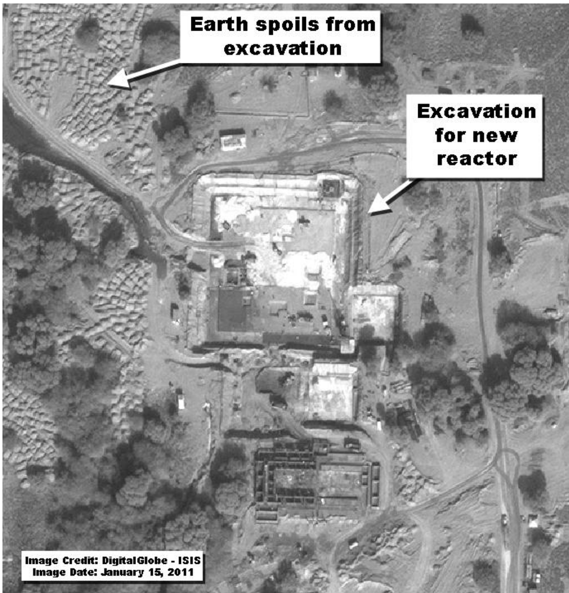
Figure 3. January 15, 2011 commercial satellite image showing excavation for the fourth Khushab reactor.
