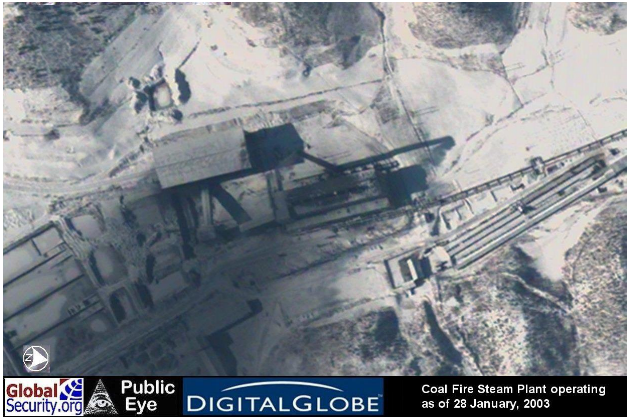
Figure 3. North Korea's coal fired steam generation plant at Yongbyon on January 28, 2003.
