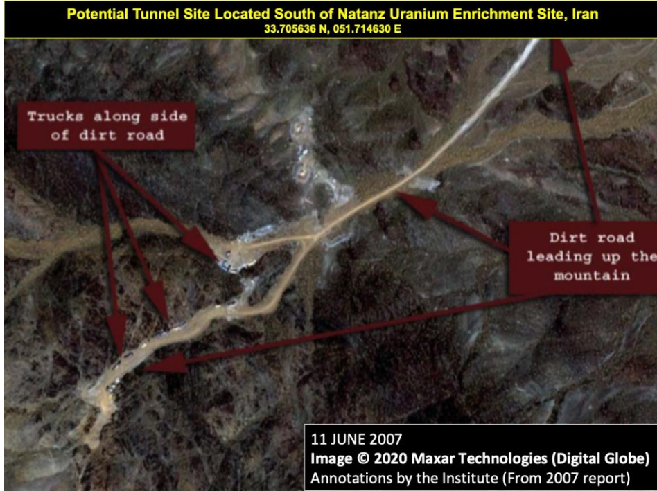
Figure 9. Area of previous construction activity in 2007 that was subsequently abandoned but now appears to have new road grading to it beginning in mid-September 2020. This image is taken directly from a 2007 Institute report.
