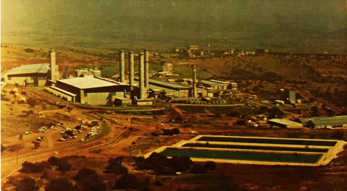
Figure 2 Y Plant, with many high stacks, with main Pelindaba site in background. The tall stacks were part of a hydrogen ventilation system aimed at minimizing the chance of an explosion of hydrogen gas used in the enrichment process lines. Photo Credit: UCOR
