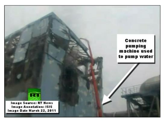
*Figure 13. Still from RT News video from March 22, 2011* showing what the Federation of Electric Power Companies of Japan describes as a concrete pumping machine pumping water into the spent fuel pool in the unit 4 building. In the video, see <u>here</u>, a plume of either steam or smoke can be seen rising from the building.
