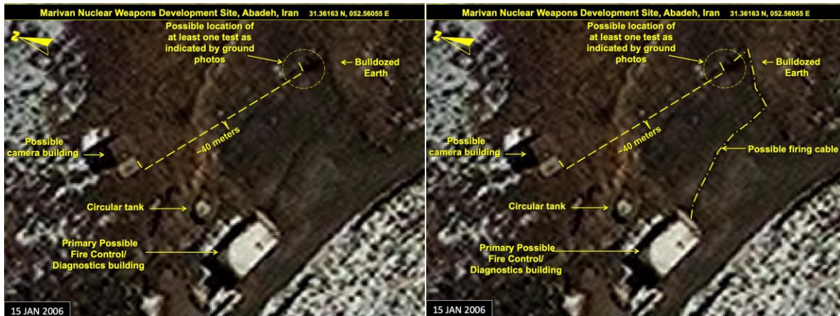
Figure 11. A January 2006 Maxar Technologies satellite image showing a possible trench for cabling running from the primary possible fire control/diagnostics building to the possible outdoor testing location.
