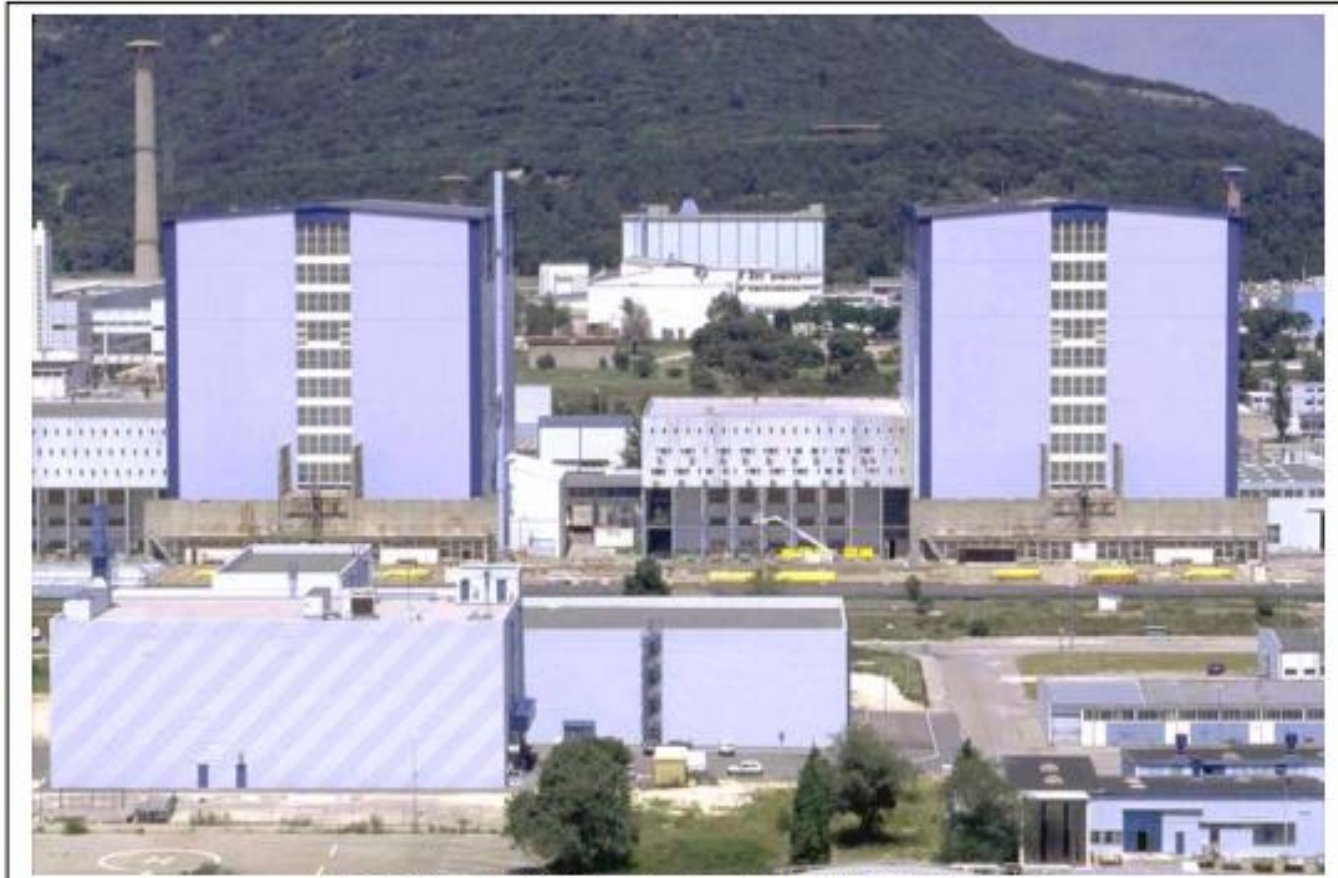
The G2 and G3 reactors on the Marcoule site
