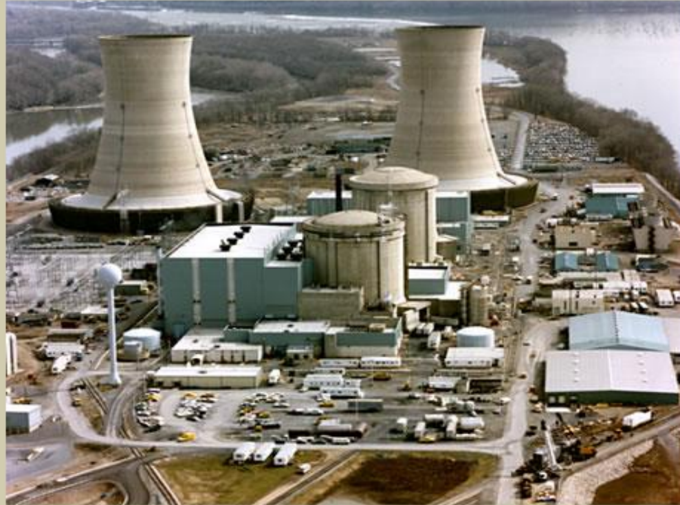
Figure 8: Three Mile Island Nuclear Power Plant. Note the domed containment silos (center) and separate fuel-containment building (left of silos) distinct to pressurized water reactors, and the natural-draft cooling towers. The reactors must be housed in these external silos rather than in the single facility used in boiling water reactors (see Figure 7) because the reactors are themselves much larger.
