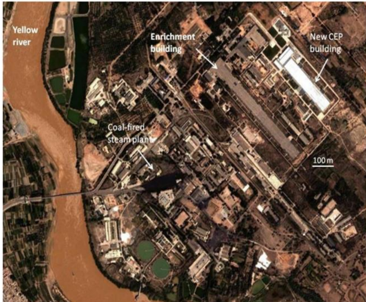
Figure 1: Lanzhou gaseous diffusion plant. Satellite image from 5 July 2004.
